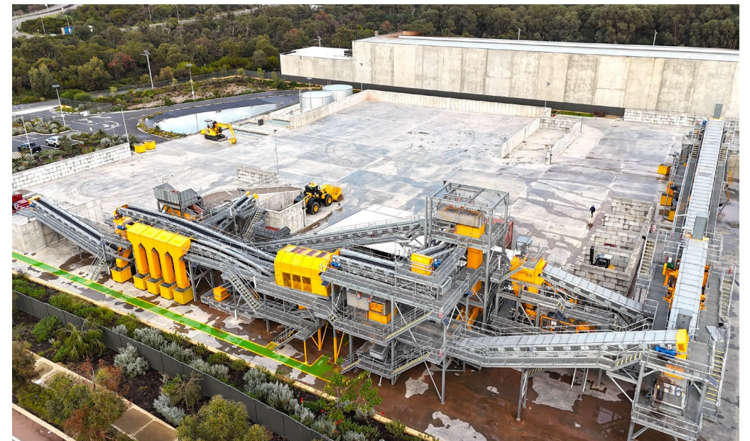
IBA PROCESSING FACILITY IN PERTH, AUSTRALIA
