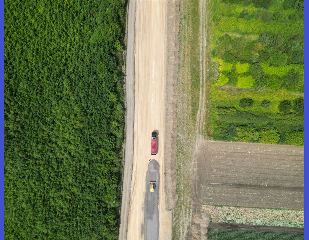
BLUE PHOENIX IBA AGGREGATES ROAD-BASE APPLICATION IN OEVERMANN, GERMANY
