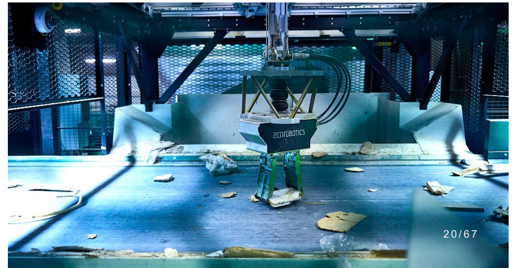
ZENROBOTICS FULLY AUTOMATED PLANT, DENMARK
